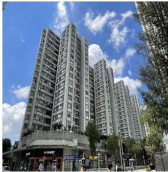
EV Infrastructure at Lei King Wan
