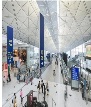
Hong Kong International Airport
