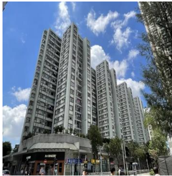
EV Infrastructure at Lei King Wan
