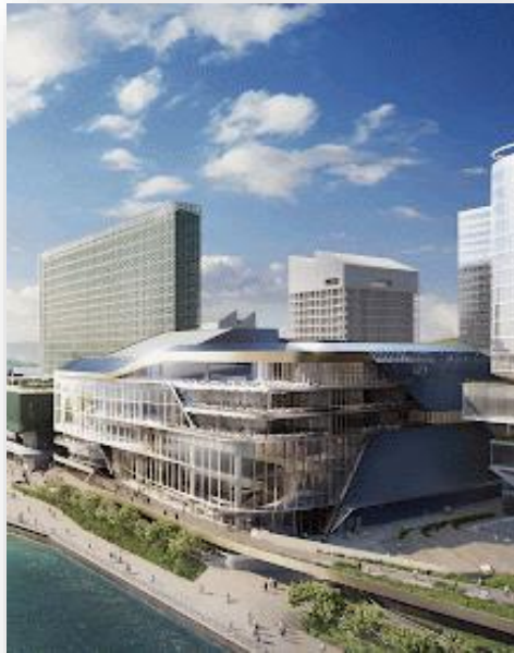
Lyric Theatre Complex Sea Water Electro-chlorination System – Environment Solutions
