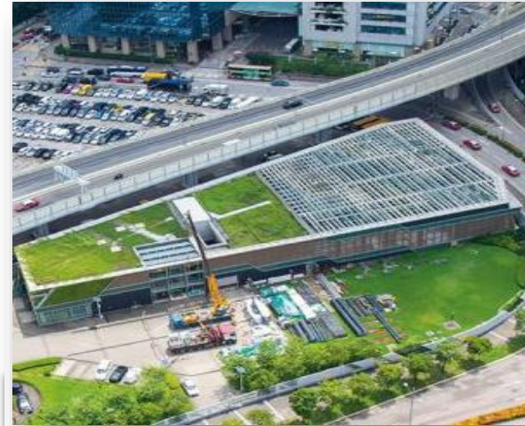
Kai Tak ADCS Sea Water Electro-chlorination System – Environment Solutions
